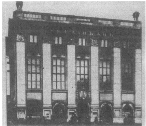
The central building of Ukrainbank in Kharkiv
