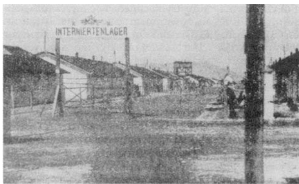
The entrance to the Thalerhof internment camp
