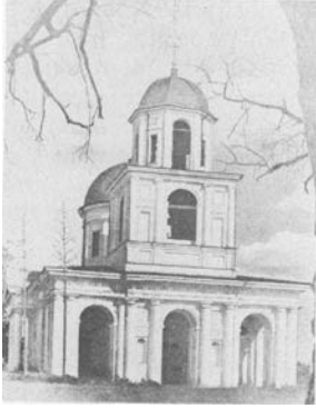
Church in Velykyi Bobryk, near Sumy, a fine example of classicism in architecture, 1808
