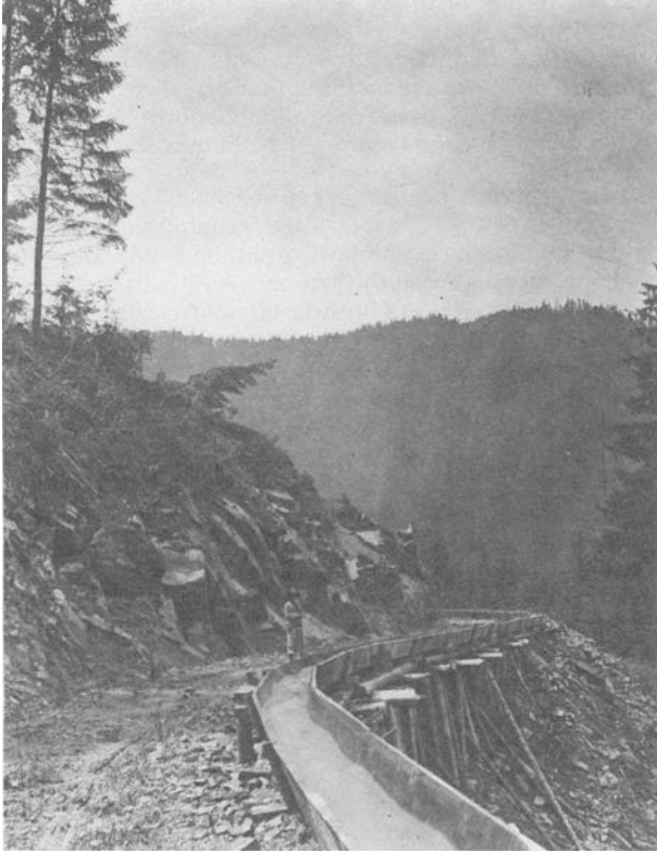
A water trough for floating logs down the mountain at the village of Hrebeniv near Stryi in the Carpathians
