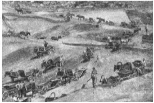
FIGURE 497. EARLY CONSTRUCTION ON THE DNEIPER HYDROELECTRIC POWER STATION (1927)
