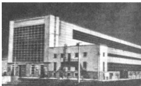
FIGURE 448. BUILDING OF A METALLURGICAL COMPLEX IN KRYVYI RIH
