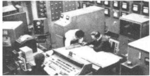
FIGURE 450. COMPUTER CONTROL ROOM AT THE AZOVSTAL PLANT
