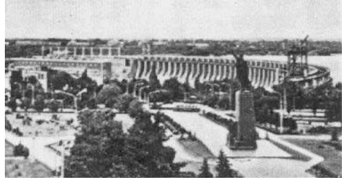
FIGURE 498. THE LENIN HYDROELECTRIC POWER STATION ON THE DNIPEP NEAR ZAPORIZHIA
