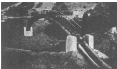
FIGURE 516. ELEVATED OIL PIPE LINE OVER THE LIATORYTSIA RIVER IN CARPATHO-UKRAINE
