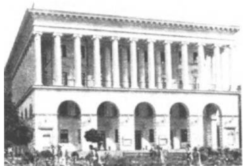
FIGURE 311. KIEVAN CONSERVATORY BUILDING
