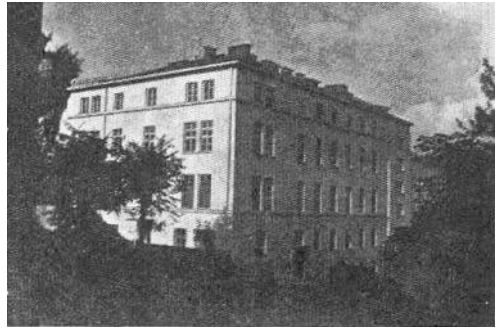
FIGURE 558. BUILDING OF THE NARODNA LICHNYTSIA HOSPITAL IN LVIV, 1937
