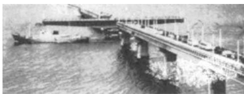
FIGURE 508. BRIDGE ACROSS THE SOUTHERN BUK RIVER IN MYKOLAÏV
