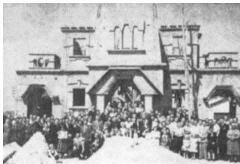
FIGURE 684. CONSTRUCTION OF A UKRAINIAN ORTHODOX CHURCH IN SÃO CAETANO DO SUL (1955)
