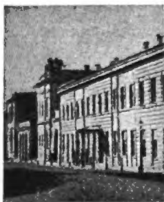
FIGURE 442. UNIVERSITY OF KHARKIV (OLD BUILDING)
