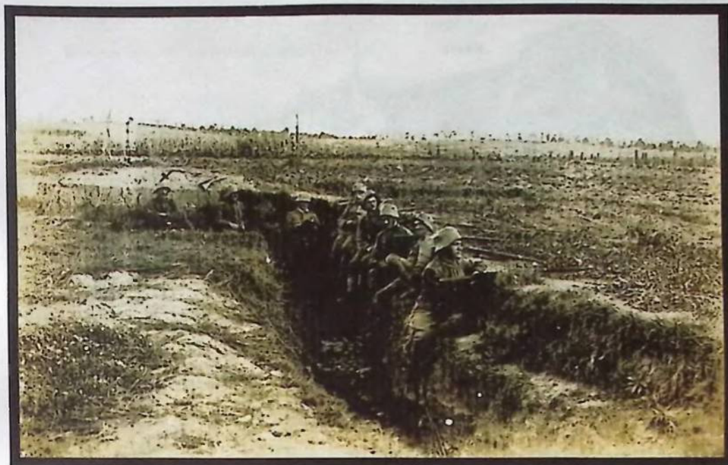
in the trench - note cross above the sender sat in the trench!
