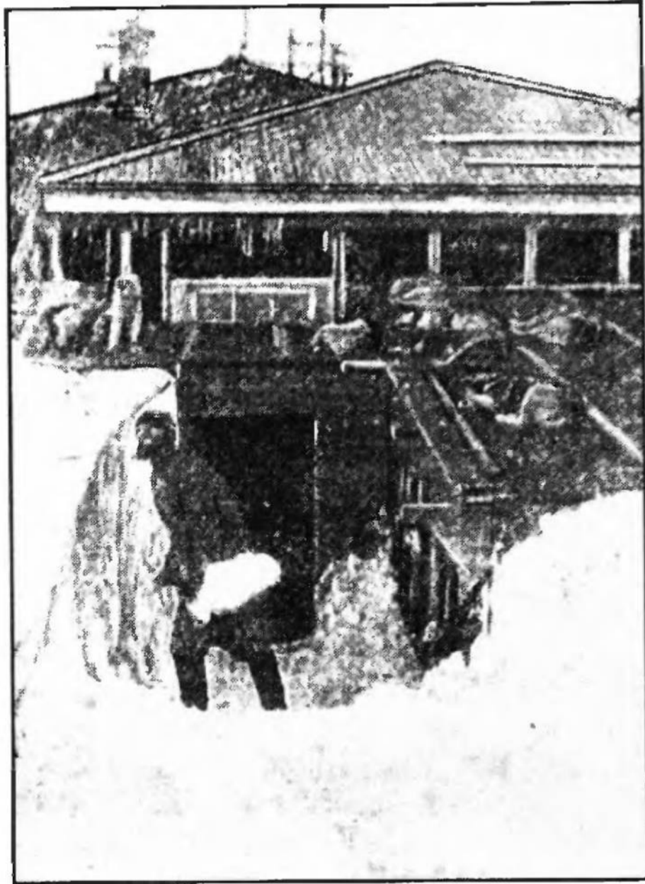
Zymovchyks clearing snow from the entrance to the station, June, 1932
