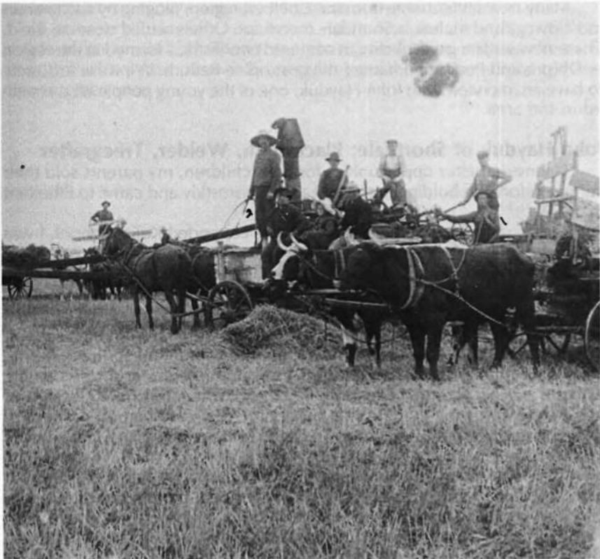
Bill Kuzyk's yoke of oxen used to haul sheaves.
