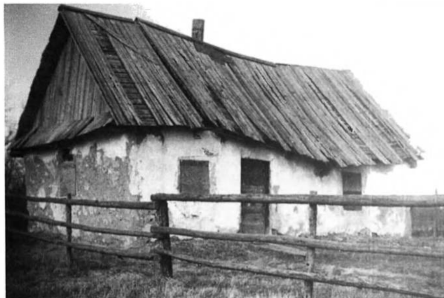
Iwan Lysyshyn home, Kosiw District c. 1908. Note type of board roofing. (W. Sklepowich Coll.)
