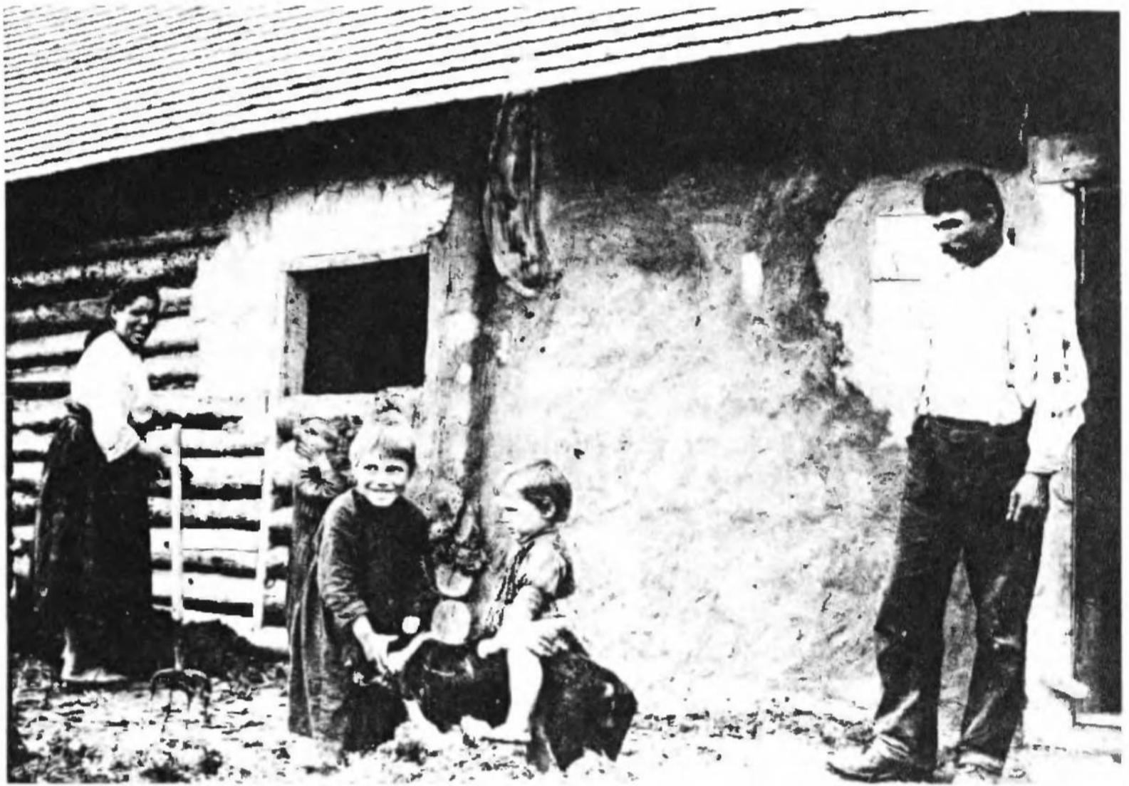
Family outside partially plastered dwelling. Both preparation and application of the plaster, primarily a mixture of clay and straw or cut slough grass, were typically women's work. Lamont, Alberta, c.1920
