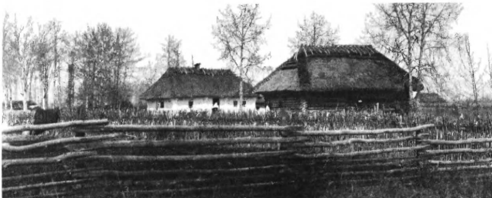
Ukrainian farm in the Vegreville bloc, east-central Alberta, late 1920s. Despite widespread replacement of traditional peasant architecture with Canadian-style buildings between the wars, the thatched and whitewashed cottage did not disappear.
