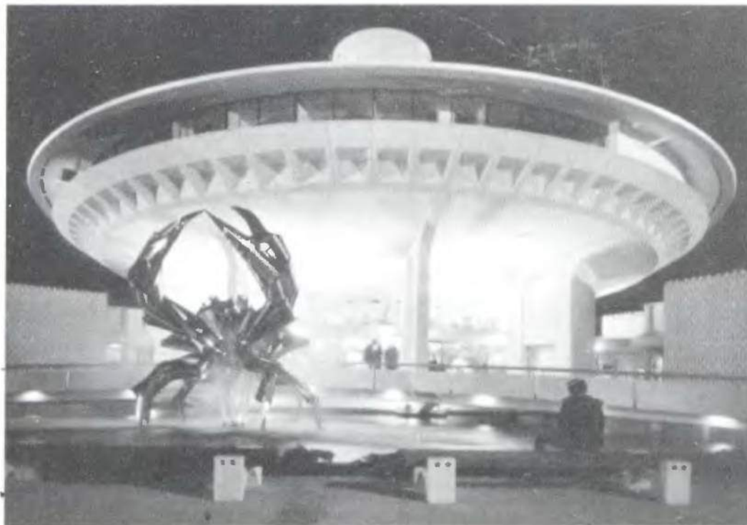
H.R. MacMillan Planetarium (a Vancouver Centennial Project).
