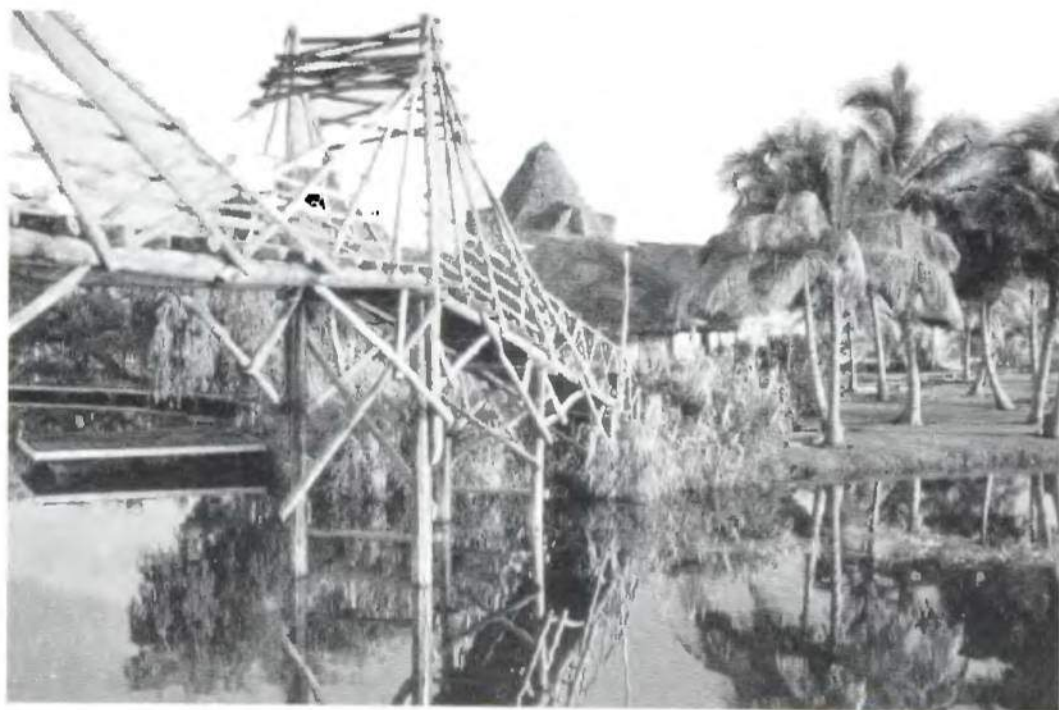
Wooden bridge at Guama.
