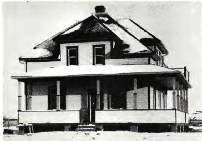
Mykola Sydor Shandro's newly built second home, 1920 (Bobersky Collection Ba48)
