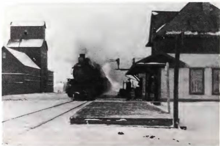
Railway station and grain elevators, Mundare, 1920 (Bobersky Collection, Oseredok, Winnipeg, Ba250)
