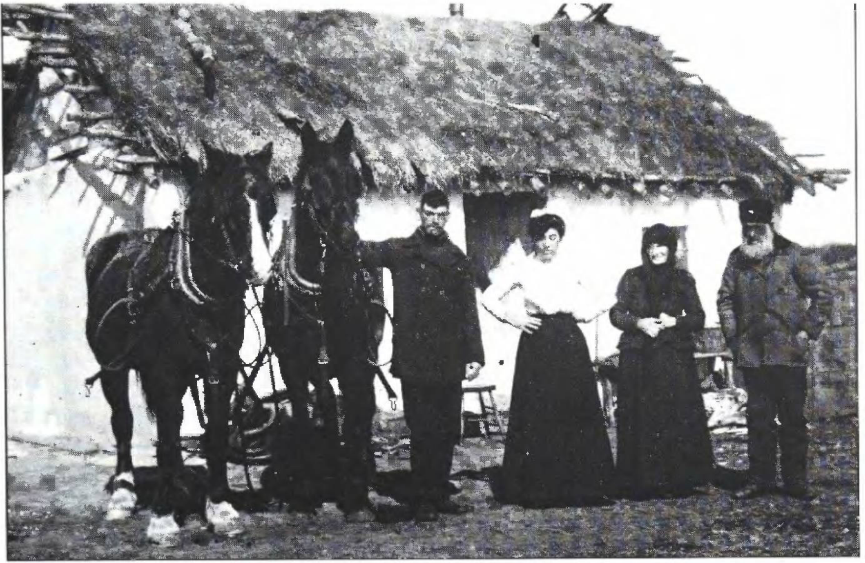
5. The first permanent home of the Ukrainians usually had a thatched roof and two rooms. The floors were packed clay, washed every week with a solution of cow dung and water. This home was built in Saskatchewan about 1903.
