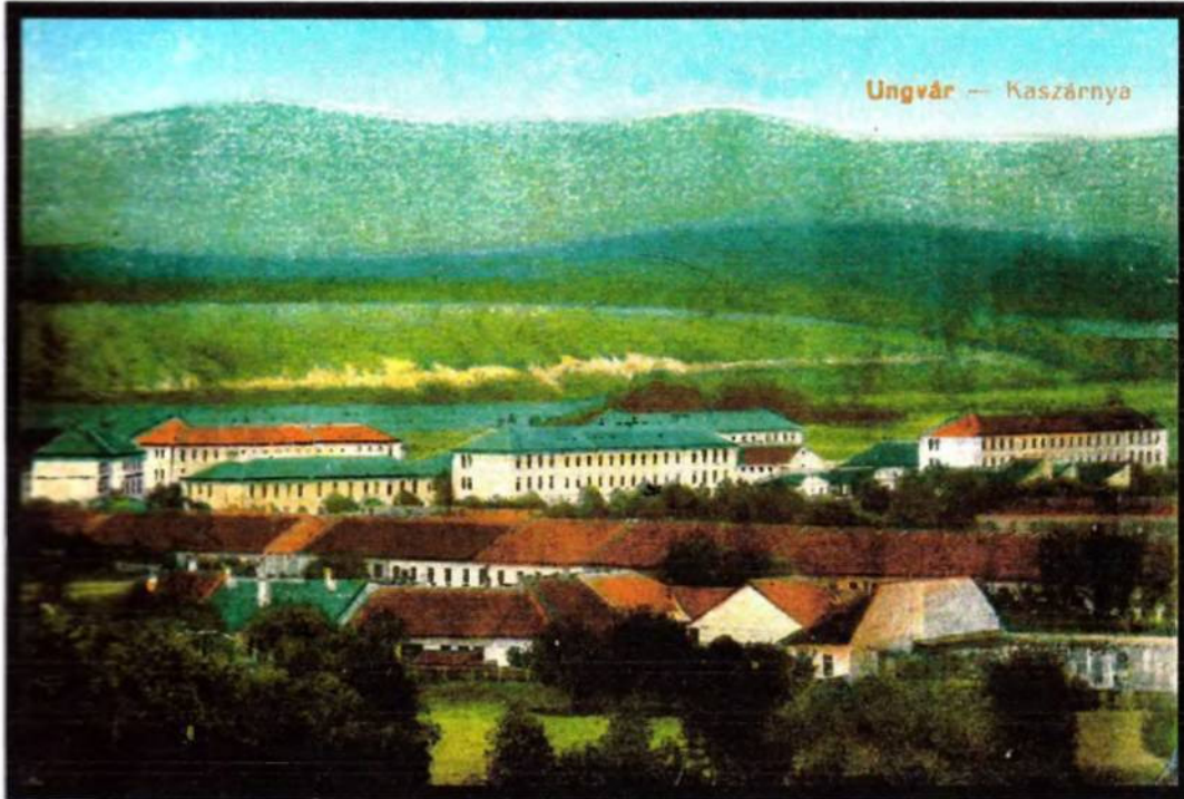
The Military Barracks in Uzhorod (U5)
