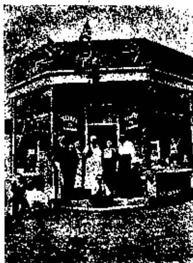
Co-operative Store "Future" in Sudbury, Ont., established in 1936. At present employs seven persons. The building valued at $9,000.00 is owned by the Co-operative.
