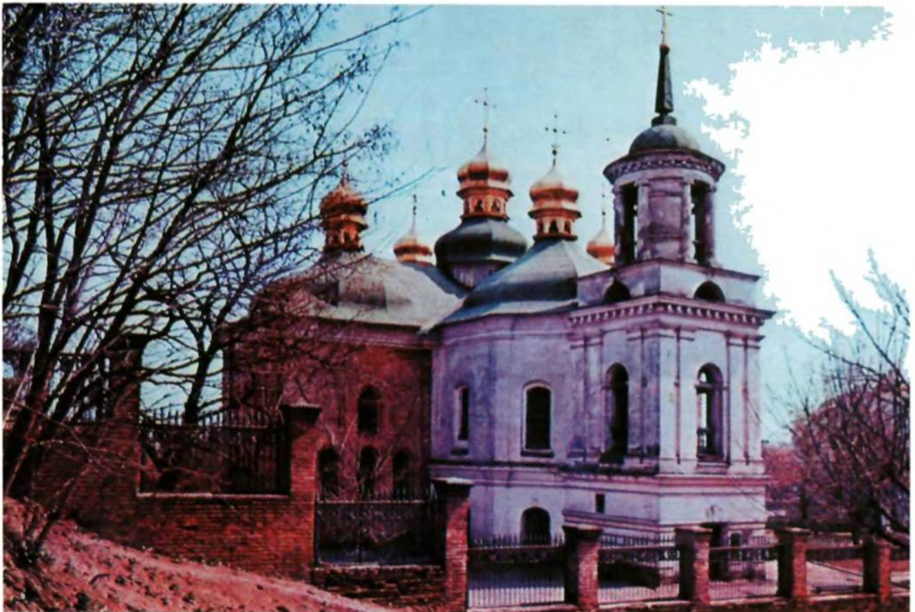
The Church of Our Saviour in Berestova- Kiev, built in the 12th century.
