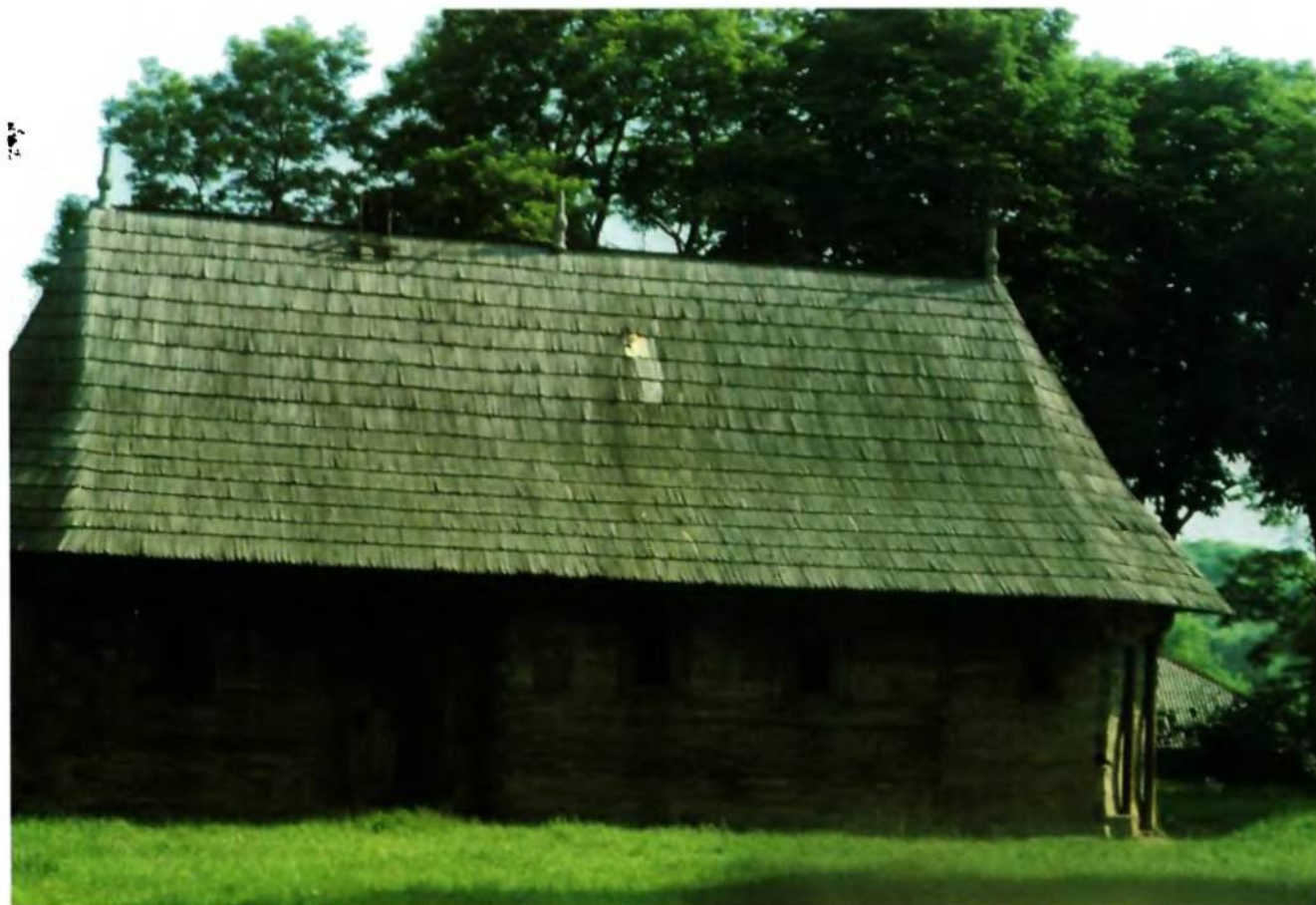
The Church of Saint Nicholas, one of the oldest wooden church in Chernivtsi, built in 1607.
