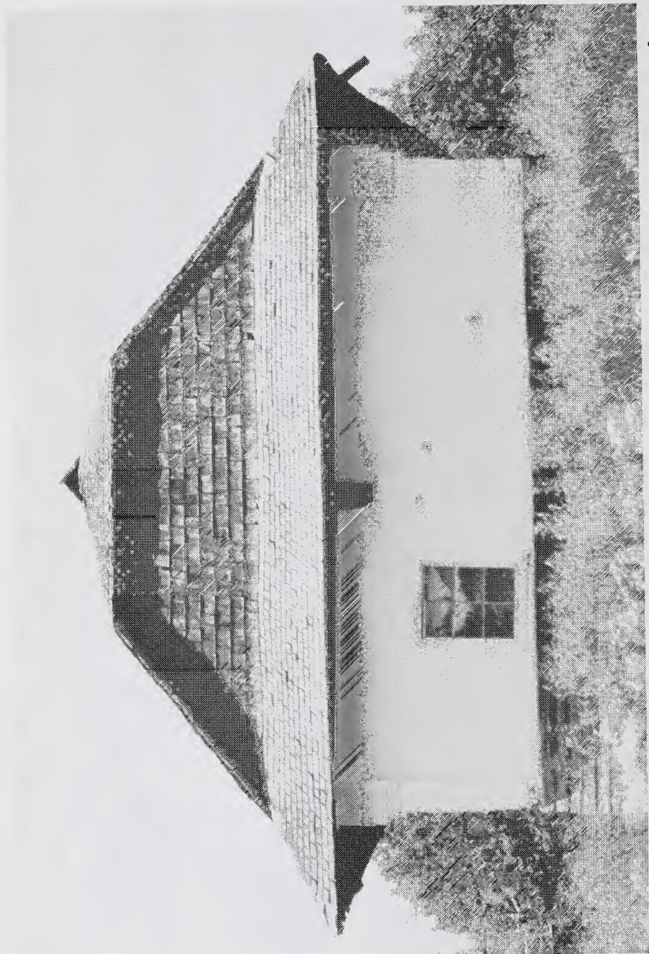
Fig. 41. The west facade of Grekul House was less affected by Alberta's prevailing westerly winds than the other facades, and was therefore in fair condition even in 1973, despite a broken pole hanging from the north-east eaves. The yard by this time was overgrown with various grasses. Photograph by Peter Shostak, summer, 1973.
