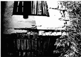
Figure 5. Dovetail jointing
