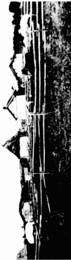
Figure 8. Galician homestead on old Athabasca Landing Trail, 1912. Note the varied roof pitch in accordance with differing roofing materials: sod roof - low pitch, shingle - medium pitch, and thatch - high pitch. (Ernest Brown Collection, Provincial Museum and Archives, Alberta.)
