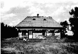
Figure 17. Bukowinian house type with hipped roof and eyebrow vents.
