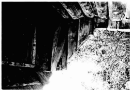
Figure 20. Eave bracket and eave detail. House of John Shandro, Shandro, Alberta
