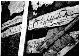
Figure 4. Shaped log. Broadaxe markings are clearly visible, also angled wood strips attached to log to provide purchase for plaster.
