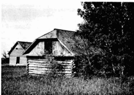
Figure 3. Inferior aspen log used in wall construction.
