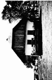
Figure 19. Bukovinian house type; extensive roof projection on southern facade.
