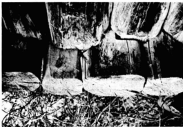
Figure 6. Notched log jointing
