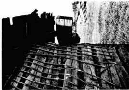
Figure 12. Willow lathes on shaped log walls
