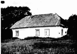
Figure 10. Bukowinian house type with hipped gable roof.
