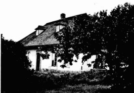
Figure 18. Modification of eyebrow vents into small dormers on a Romanian style house, Sandy Lake, Alberta.
