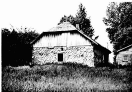
Figure 11. Wood lathes attached to shaped logs afforded purchase for mud plaster.
