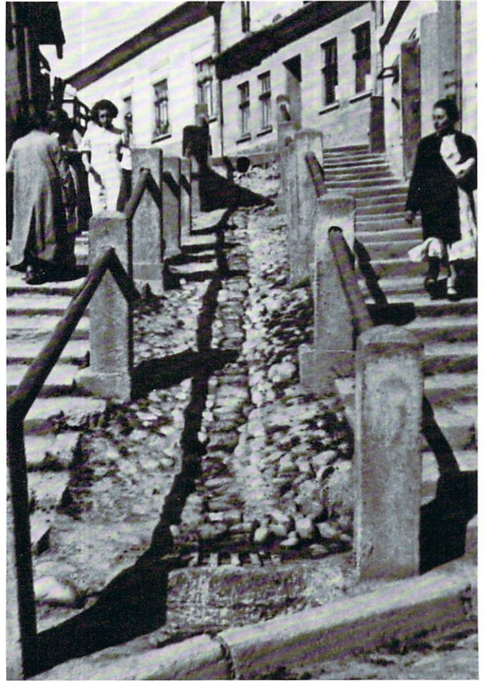
A curious piece of canalization on a downtown Kolomiya street. Dirty water ran openly along the section of the street with an outlet pipe at the top and an inlet pipe on the bottom.
