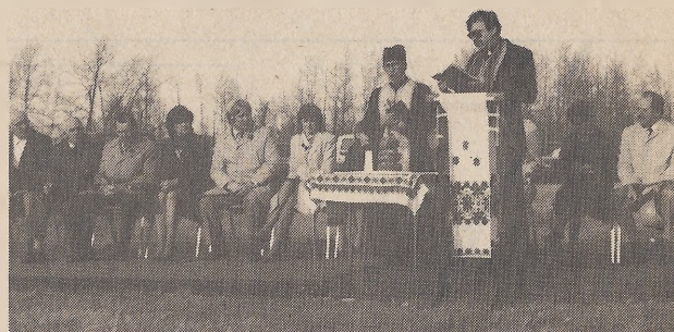
Blessing of site - November 5, 1983.
