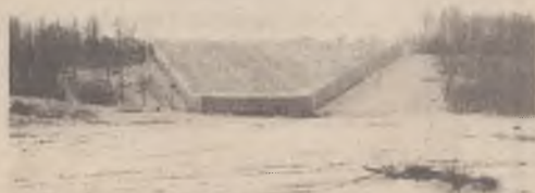
Building hoarding for winter construction of amphitheatre - January 1984.
