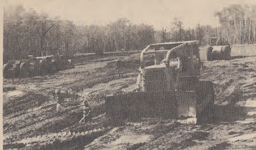
Preparing slope for amphitheatre - November, 1983.
