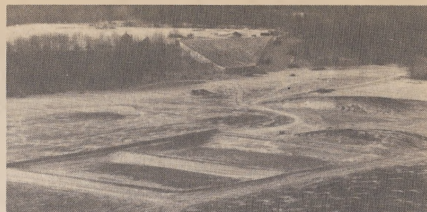
Construction of lagoon completed - December, 1983.
