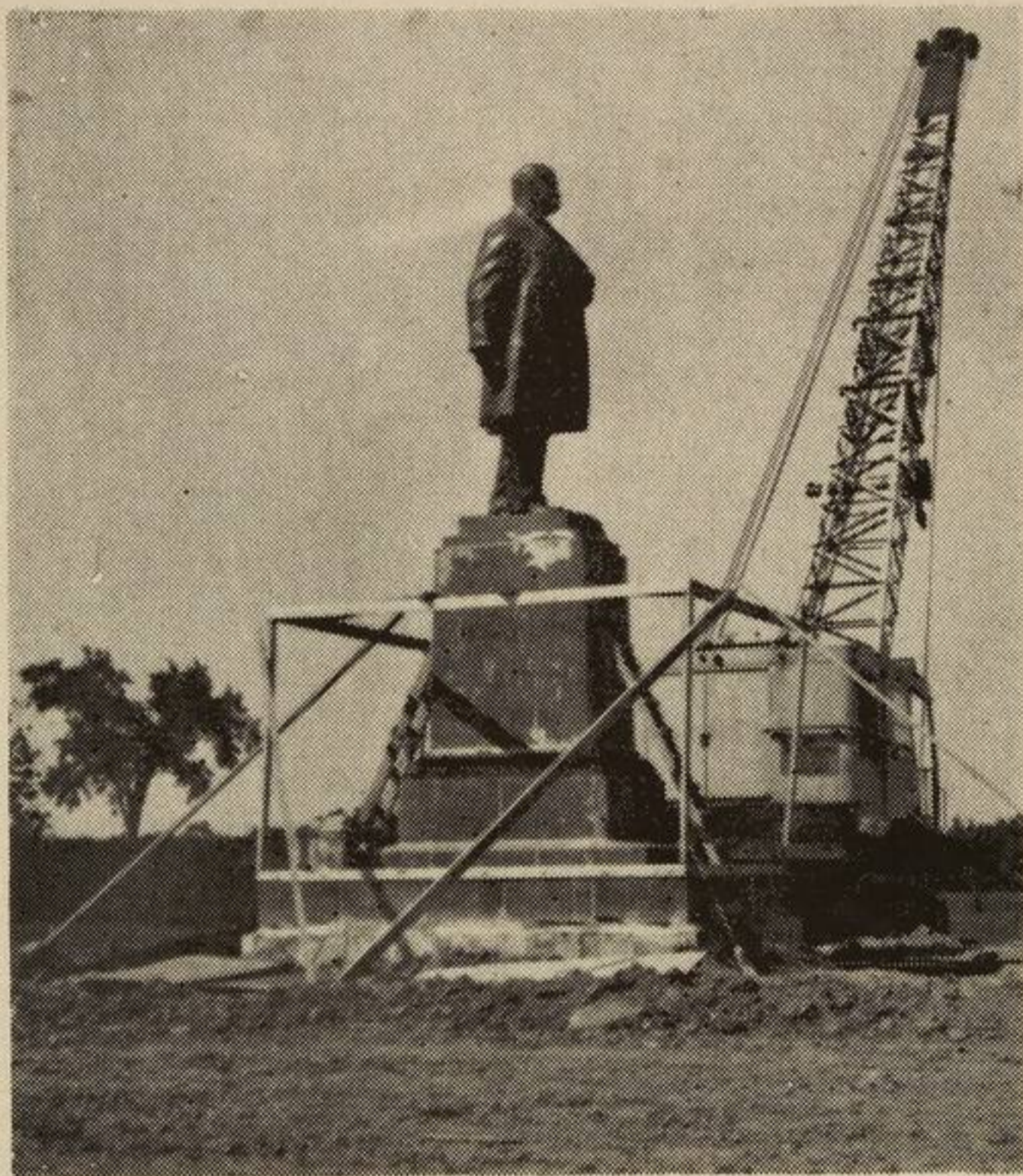
The Shevchenko monument at Palermo just after the mighty crane had lifted it up to its pedestal (a single 10½ ton piece of granite). The statue itself is in bronze and weighs seven tons. This year, 1961, marks the 10th anniversary of the unveiling of the statue at Shevchenko Park in Palermo.
