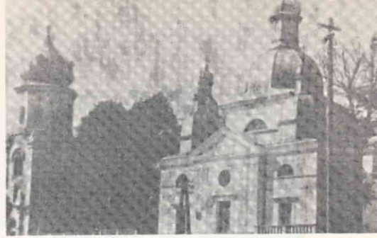
Ukrainian Catholic church of the Redemptorist Fathers in Ternopil, demolished by the authorities in the summer of 1962.
