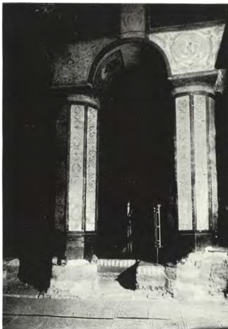
Columns of the triple arch structure in the northern part of the transept (ground floor level). Here, the floor was lowered to its 11th century level in 1939.
