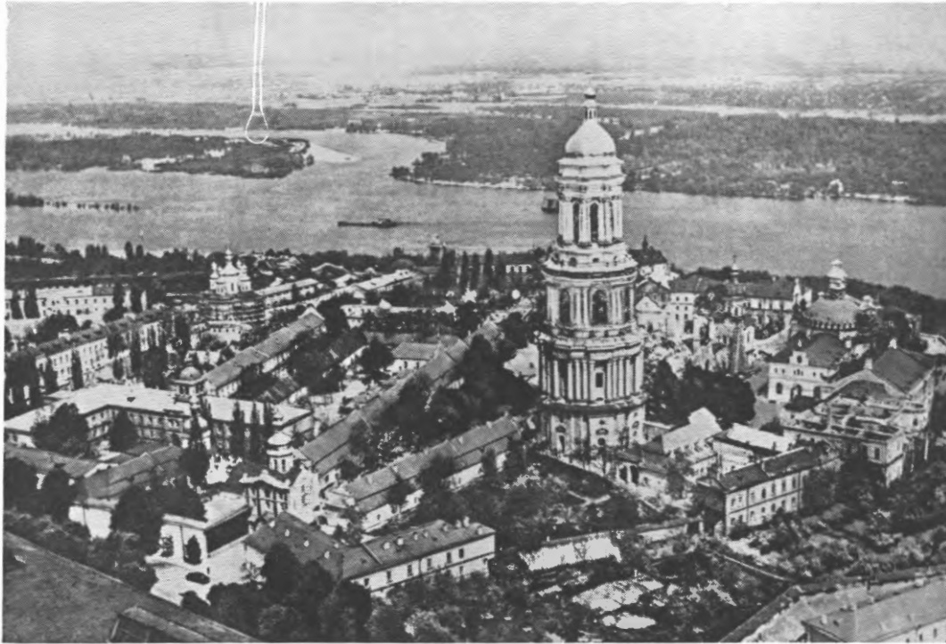
THE MONASTERY OF THE CAVES IN KYIV (Pecherska Lavra), the most venerable in Eastern Europe, dating back to the 11th Century. A part of it has been transformed by the Bolsheviks into an anti-religious museum, and its main monument, the Church of the Assumption, seen on the right, was mined and blown up by them in 1941, during World War II.
