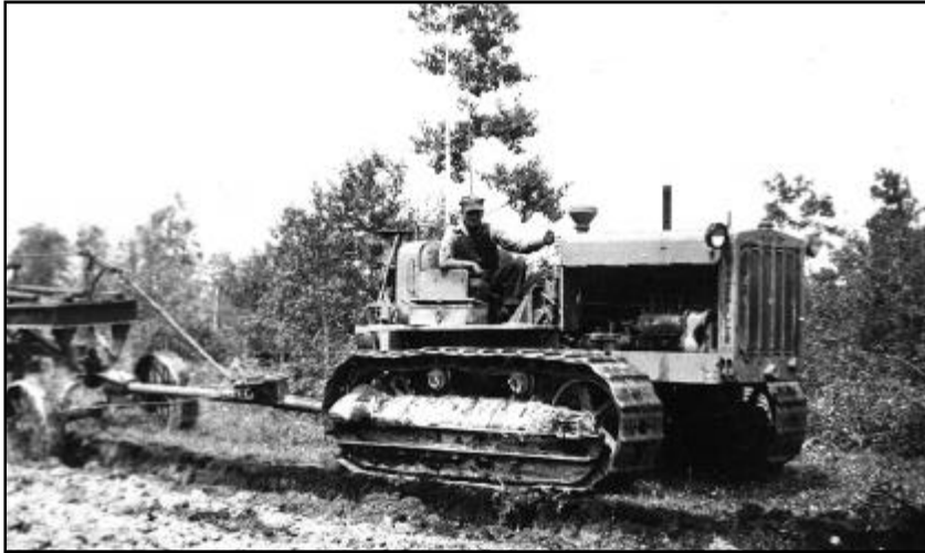
Above and right: On higher ground, during the 1940s the dragline was not required for digging out the ditches for roadbed material. The job was normally done using a caterpillar and large four-wheeled scraper such as the one photographed in operation building up PTH#17 south of Poplarfield on July 7, 1942. RTM-068, RTM-069.
