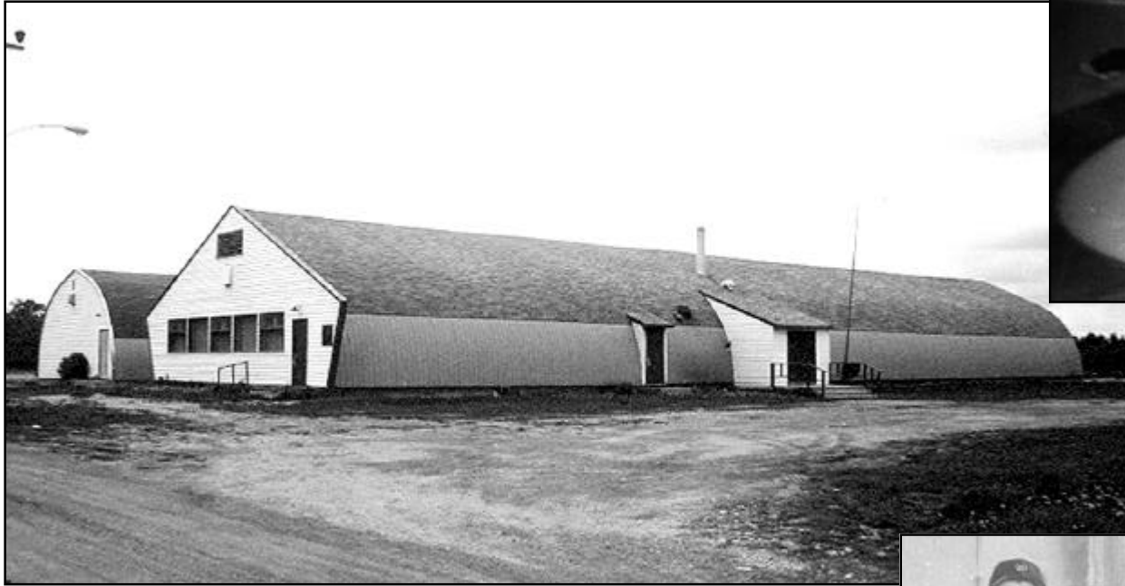
Poplarfield Community Centre and Curling Rink in 1992. CL-108.
