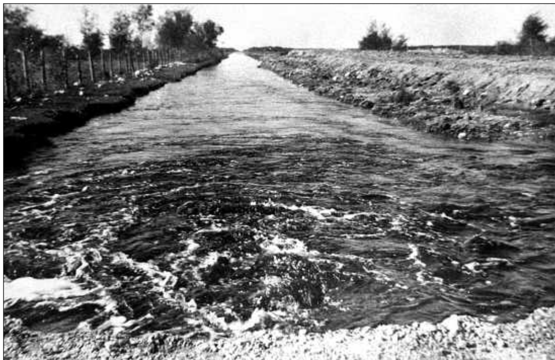
Left: Spring runoff in the newly enlarged Buffalo Lake drain where it passes under PTH #68 two miles east of Poplarfield. Late 1950s. RTM-031.
