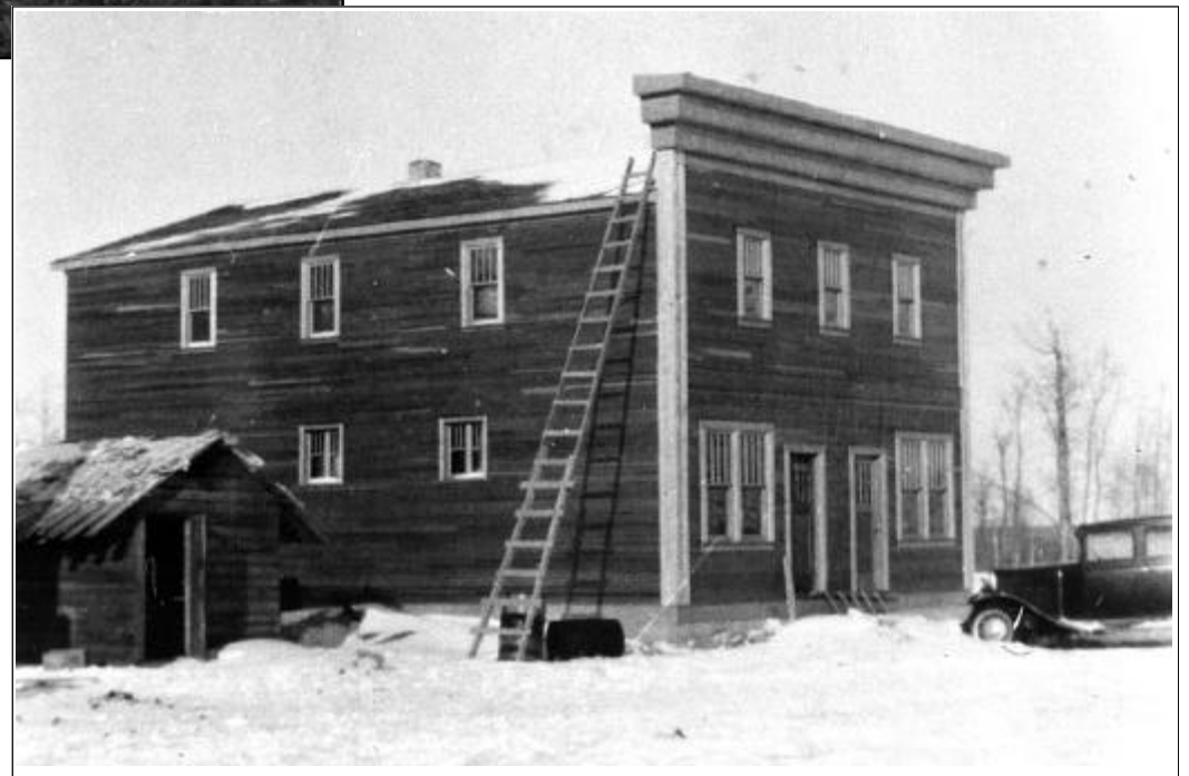
Right: The Coronation Hotel in the 'new' Poplarfield townsite, as it appeared shortly after its construction during the winter of 1938-39. The Coronation Hotel was the second building to be constructed in New Poplarfield. It was built for Steve and Mary Chreptyk, who at the time were in partnership with Walter and John Chimchak. John and his wife operated a store in the adjacent lot. CL-048.
