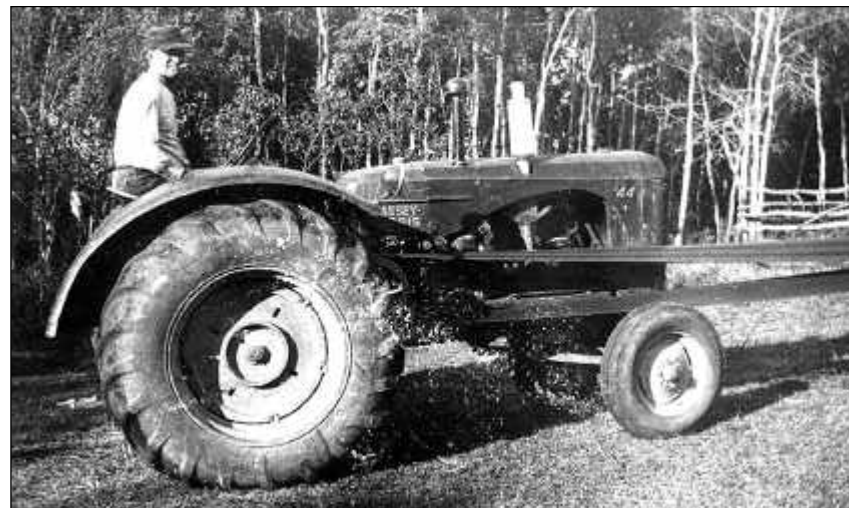
Above: Panko Zazitko running a belt-drive from his Massey-Harris tractor. By the early 1950s most of the steel wheeled tractors were being replaced by models on rubber tires. FL-127.
