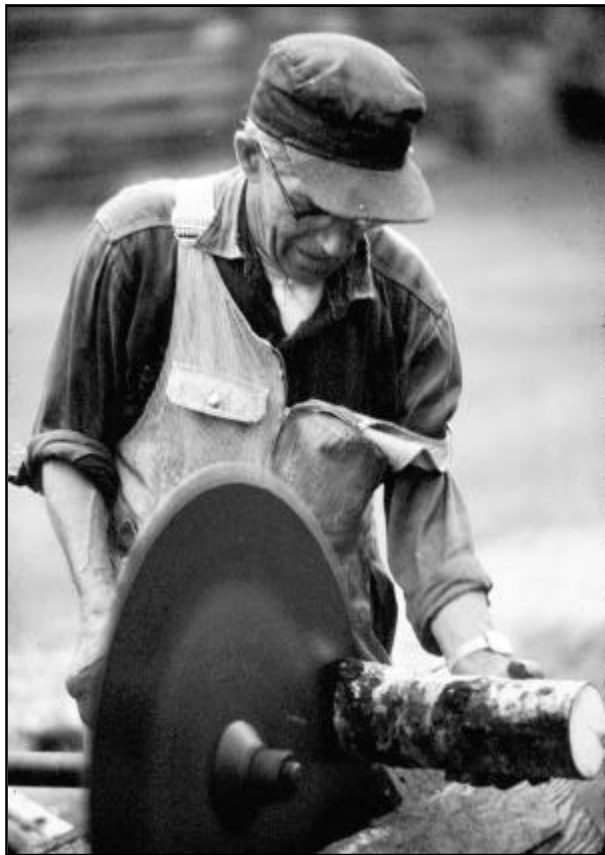
Bill Pawluk sawing firewood with a one-cylinder stationary engine, by himself. Sawing firewood with a rip-saw is a difficult and dangerous job for one person. Here Bill, at 68 years of age, has managed to rip a large pile of firewood without assistance, as winter fuel for his little retirement house which he shared with brother Andrew. Circa 1973. RTM-038 to RTM-041.
