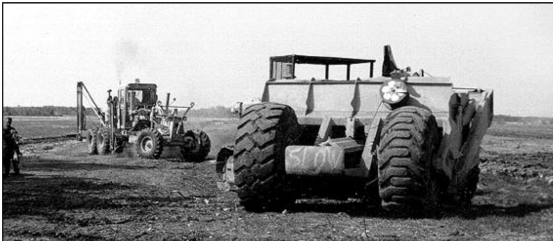
Above: By the 1960s and 1970s road building equipment had increased in both size and efficiency, and more and more of the farmyards in the region were connected to the 'main roads' with proper all weather section roads. Tom Ledochowski, son of Hamrluk pioneer Mike Ledochowski, owned a small road building operation and built many of the section roads in the region. He was photographed here in 1970 checking his crew as they worked on a job near Poplarfield. RTM-067.
