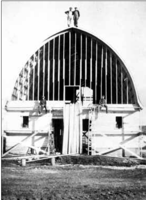
Above: Mr. John Zasitko and his wife, Pearl, are having a barn built by Mike Troschuk with the help of their sons, Fred and Bill. Bill Zasitko and carpenter Mike Troschuk standing on top of the barn, Fred and Peter Zasitko are on the lower level. The barn was completed in 1945. The loft of this barn was the scene of a number of rollicking barn dances during the late 1940s. The John Zasitko farm was situated five miles west of Poplarfield. FL-136.
